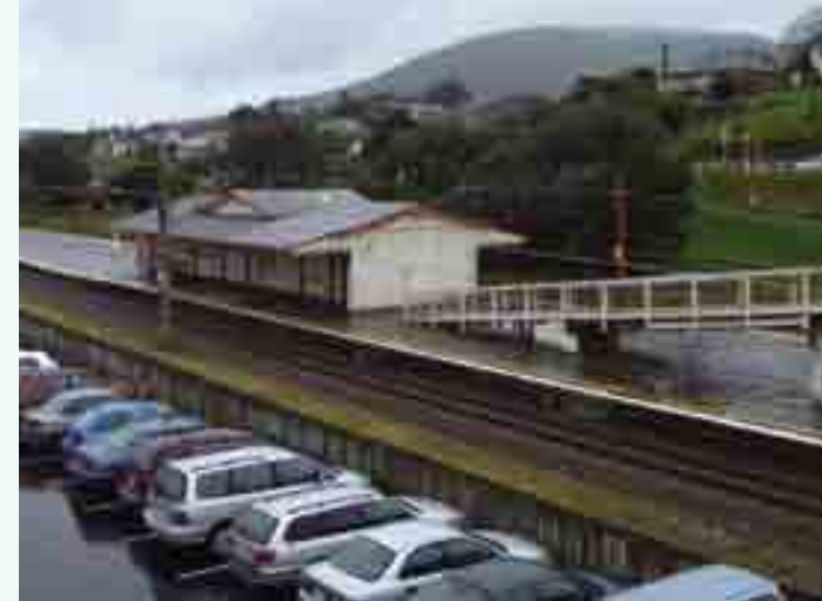
Above: Tawa Station before remedial work starts.
