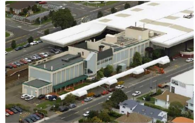
Figure 3 Waterloo Water Treatment Plant (source: WWL)
