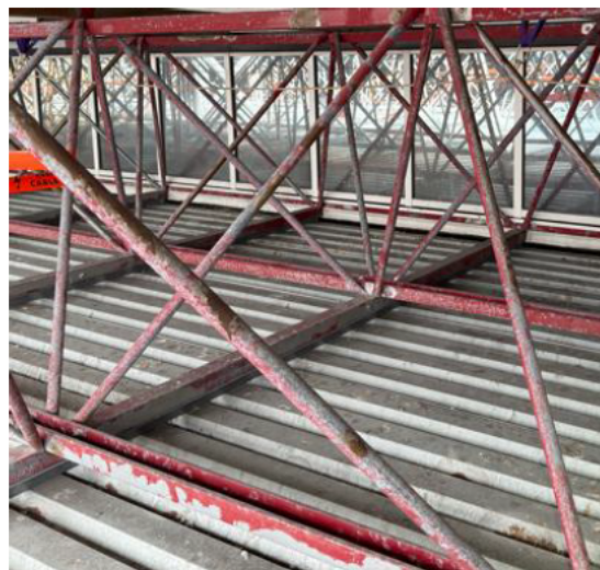
Photo 006 – Truss diagonal. Corrosion score 3.
