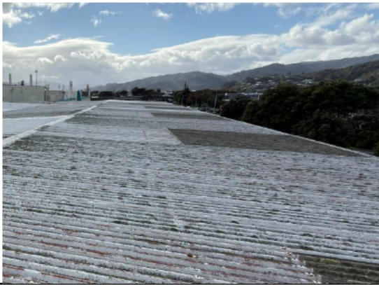
Photo 003 – Internal Gutter corrosion score 2. Water ponding was observed on the southern side of the station.
