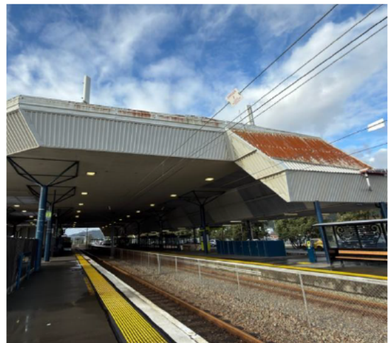
Photo 018 – Roof sheeting at Southern side of the station. Corrosion score 4.
