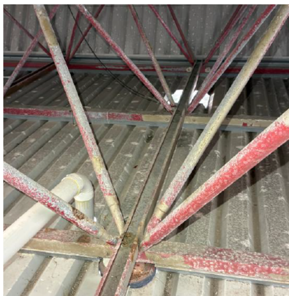
Photo 007 – Bottom Chord and Diagonals (Truss Level).
