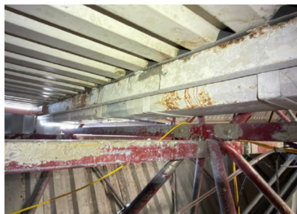
Photo 012 – Paint at the roof sheeting flaked off.
