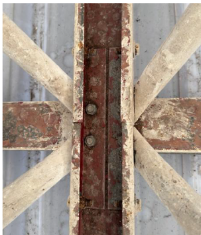
Photo 003 – Truss Bottom chord. Corrosion score 4.
