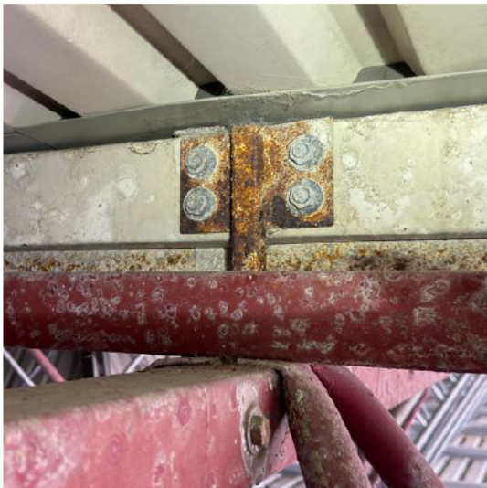
Photo 005 – Purlin Vertical Support Post northern side. Corrosion score 4.
