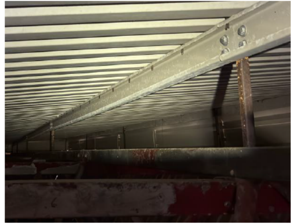
Photo 004 – Purlin Vertical Support Post. Corrosion score 4.
