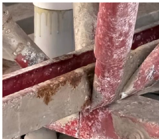
Photo 004 – Truss Bottom chord. Corrosion score 4.
