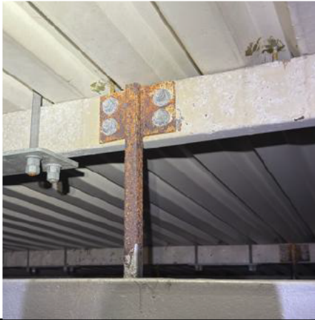
Photo 009 – Purlin Vertical Support Post lower roof northern side. Corrosion score 4.
