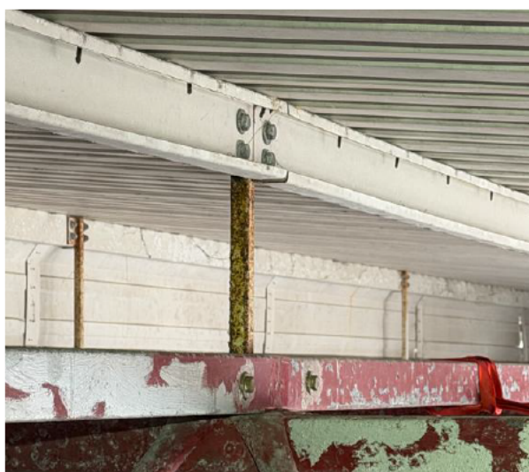
Photo 005 – Purlin and SHS Support onto Top Chord.
