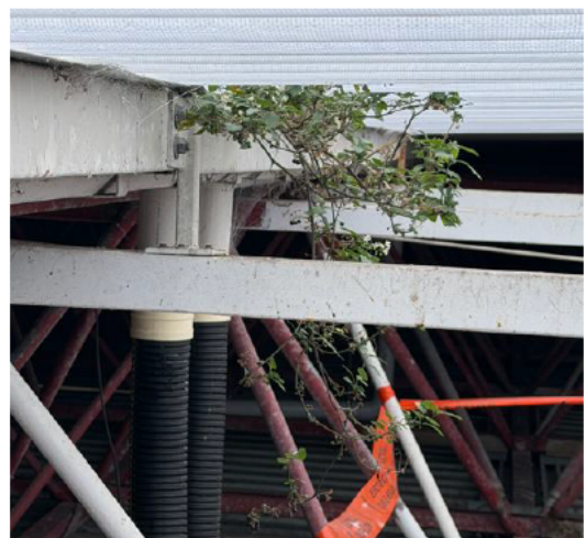
Photo 024 – Vegetation growth was observed in one area on the western side.
