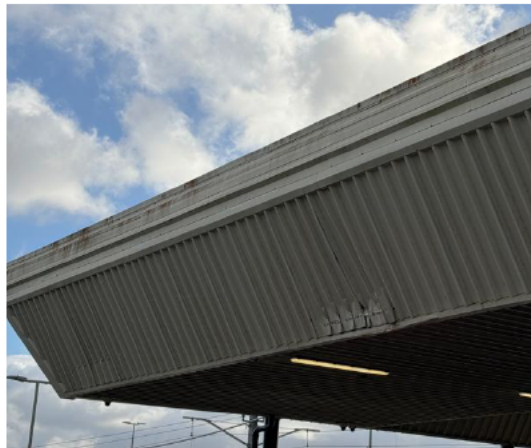
Photo 023 – Heavy corrosion at hold down screws connecting the roof sheeting to the purlins. Corrosion score 4.
