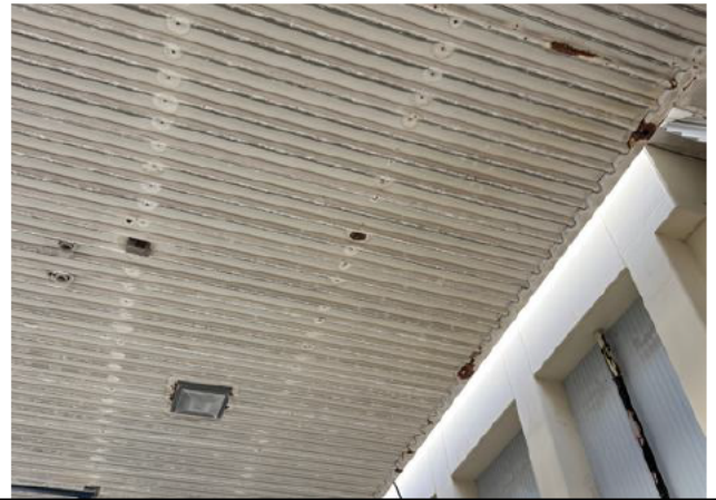
Photo 022 – Damage to the roof sheeting on the Eastern side of the station.
