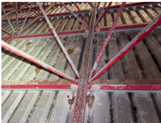
Photo 015 – Corrosion at the bottom roof sheeting (Truss Level) between GL 4-6/ GL C-D. Corrosion score 4.
