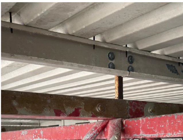
Photo 023 – Heavy corrosion at hold down screws connecting the roof sheeting to the purlins. Corrosion score 4.
