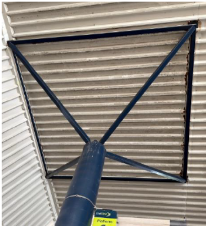
Photo 015 – Corrosion at the bottom roof sheeting (Truss Level) between GL 4-6/ GL C-D. Corrosion score 4.
