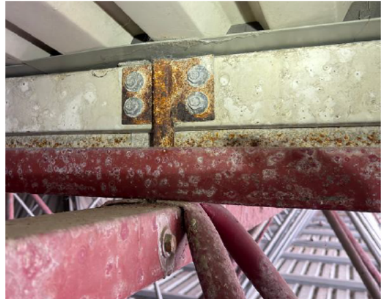
Photo 004 – Purlin corrosion. Corrosion score 4.
