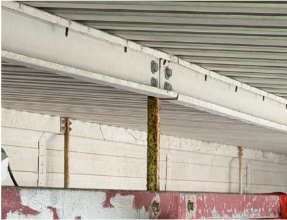
Photo 005 – Purlin Vertical Support Post northern side. Corrosion score 4.
