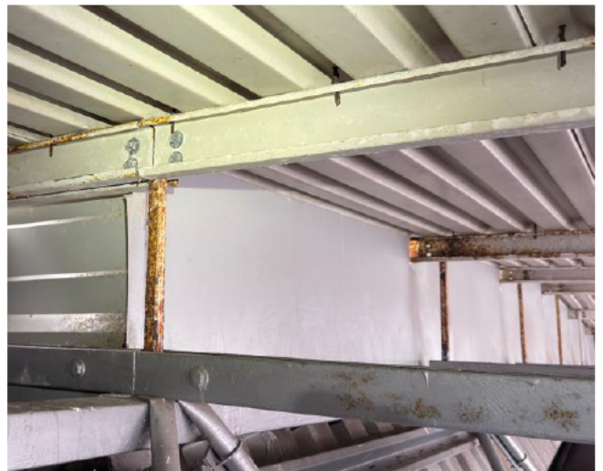
Photo 006 – Purlin Vertical Support Post northern side. Corrosion score 4.
