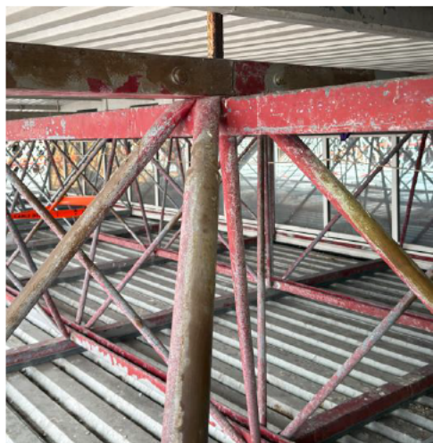
Photo 003 – Grease was applied to truss diagonal to help with the corrosion.
