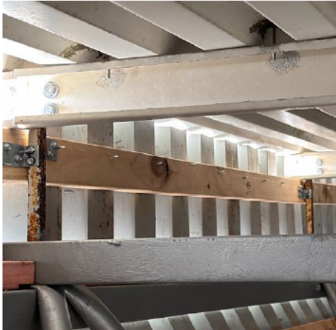
Photo 009 – Purlin Vertical Support Post lower roof northern side. Corrosion score 4.
