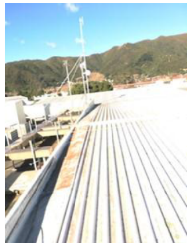
Photo 006 – Roof seismic joint corrosion score 3. Photo is from 2024 site inspection. No access to that side of the building at the time of inspection.
