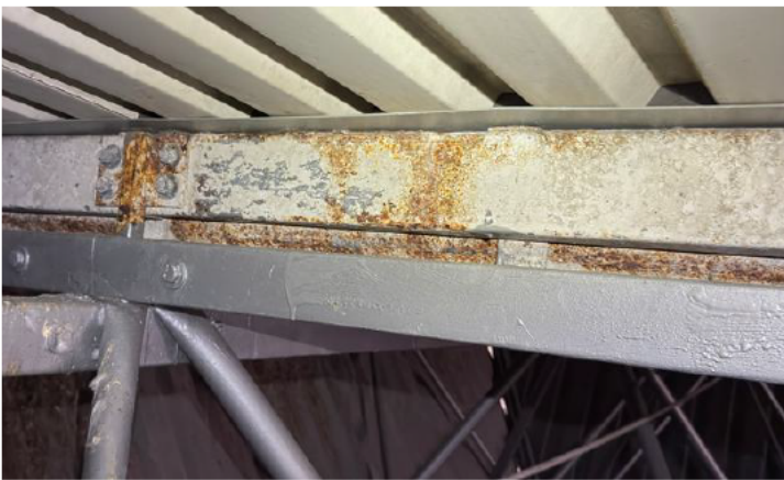
Photo 005 – Purlin corrosion. Corrosion score 4.
