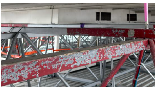
Photo 006 – Truss Top chord corrosion. Corrosion score 3.
