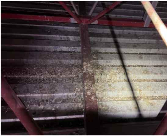
Photo 029 – Pigeon droppings at the lower roof on the eastern side.
