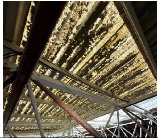
Photo 028 – Pigeon droppings on the diagonals.
