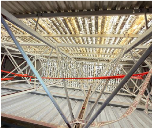
Photo 027 – Pigeon droppings observed in Truss level.
