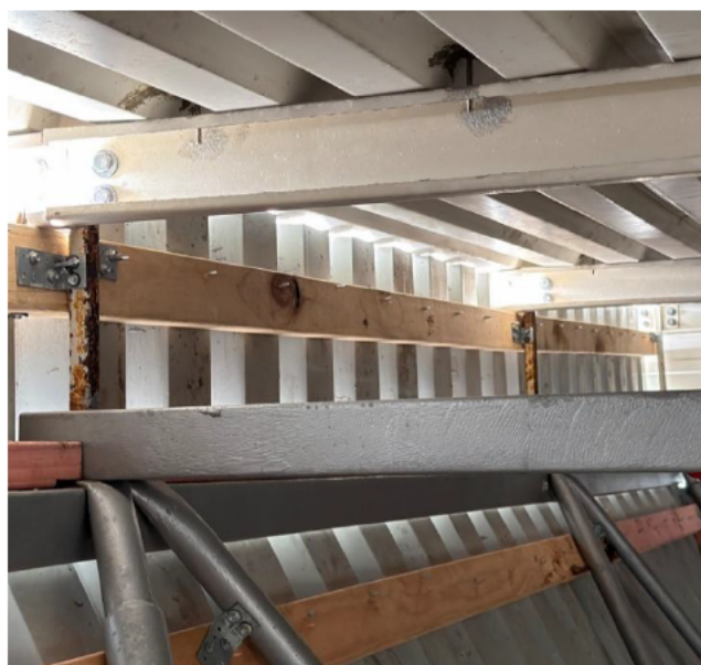
Photo 010 – Purlin vertical support (Lower Roof Level North side near Ticketing office).
