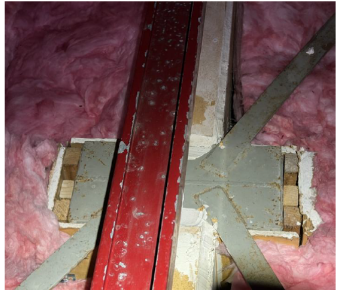
Photo 012 – Roof Bracing (Amenities Building/Bus building).
