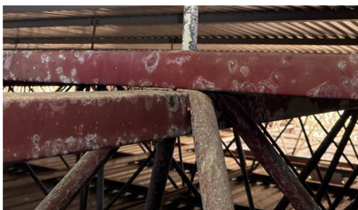
Photo 003 – Truss Top chord. Corrosion score 4.
