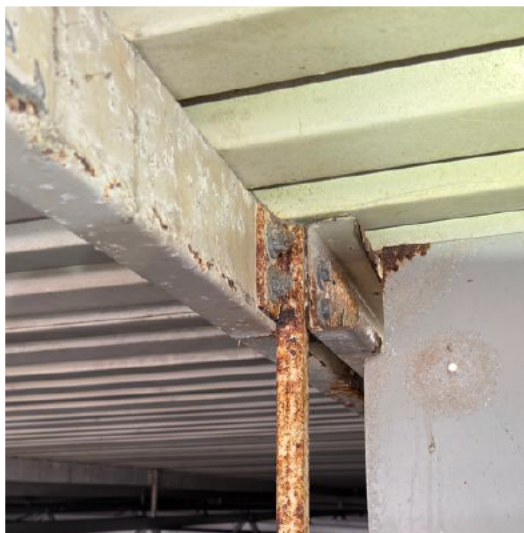
Photo 005 – Purlin corrosion. Corrosion score 4.
