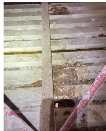
Photo 018 – Roof sheeting at Southern side of the station. Corrosion score 4.
