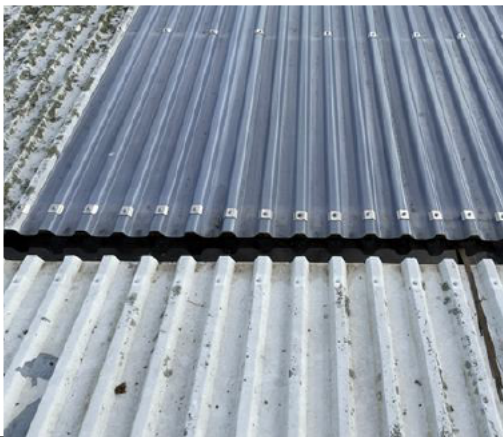
Photo 005 – Ridge capping at roof level corrosion score 2.
