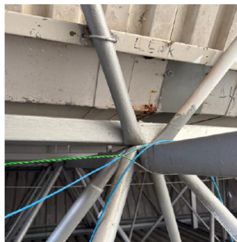
Photo 010 – Corrosion at lower internal gutter. Corrosion level 4.
