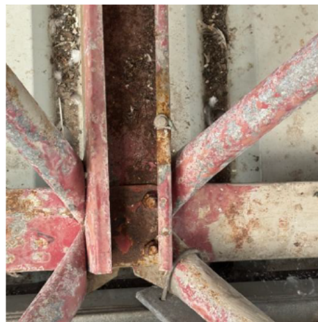
Photo 004 – Truss Bottom chord. Corrosion score 4.
