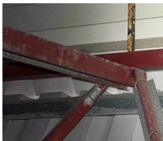
Photo 006 – Truss Top chord corrosion. Corrosion score 3.
