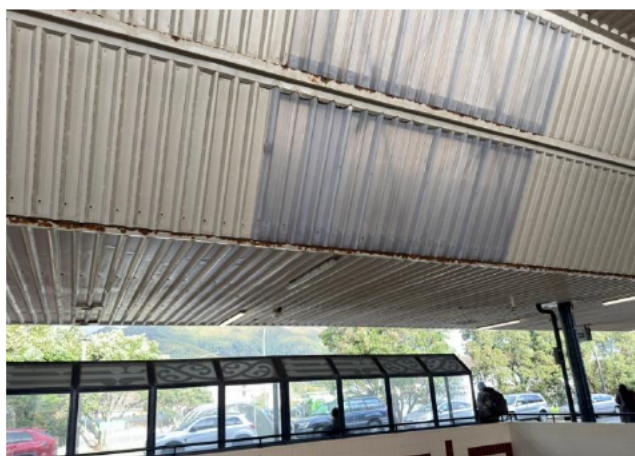
Photo 011 – Corrosion at intersection of upper and lower roof due to flashing at the corner. Corrosion level 4 on East side of the station.
