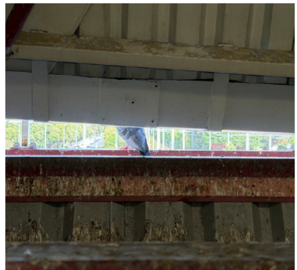
Photo 030 – Pigeon droppings at the lower roof on the eastern side. Opening for birds to enter the roof.
