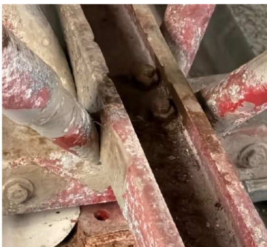
Photo 005 – Truss Bottom chord. Corrosion score 4.
