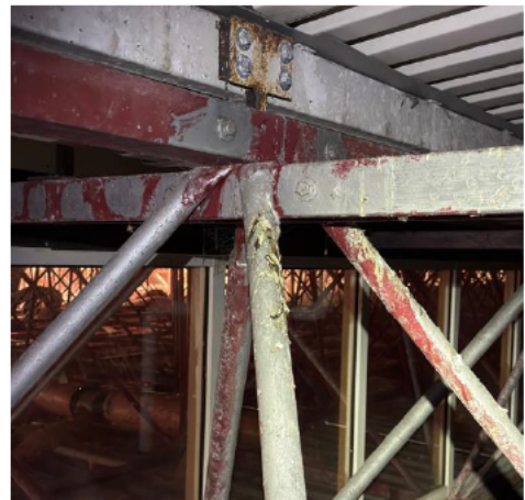
Photo 030 – Pigeon droppings at the lower roof on the eastern side. Opening for birds to enter the roof.
