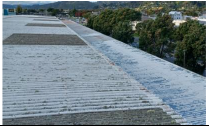
Photo 004 – Heavy presence of moss on the roof sheeting and roof walkway was observed mostly on the southern side.
