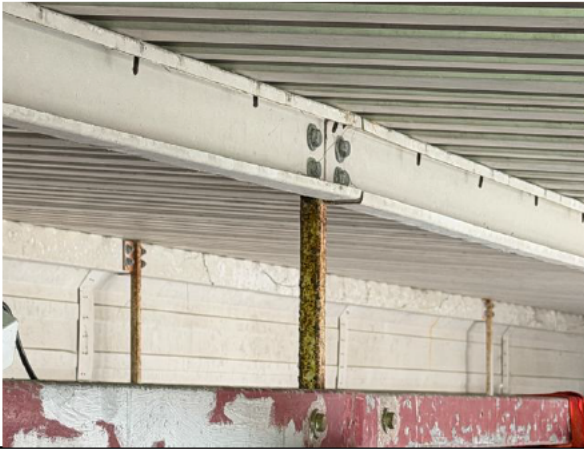
Photo 003 – Purlin Vertical Support Post. Corrosion score 4.
