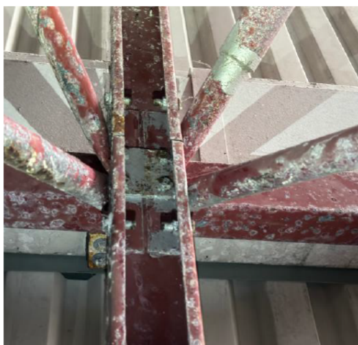
Photo 005 – Truss Bottom chord. Corrosion score 4.
