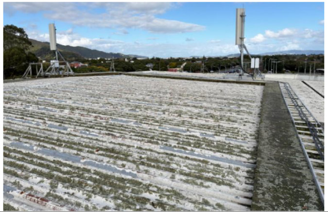
Photo 006 – Roof seismic joint corrosion score 3. Photo is from 2024 site inspection. No access to that side of the building at the time of inspection.
