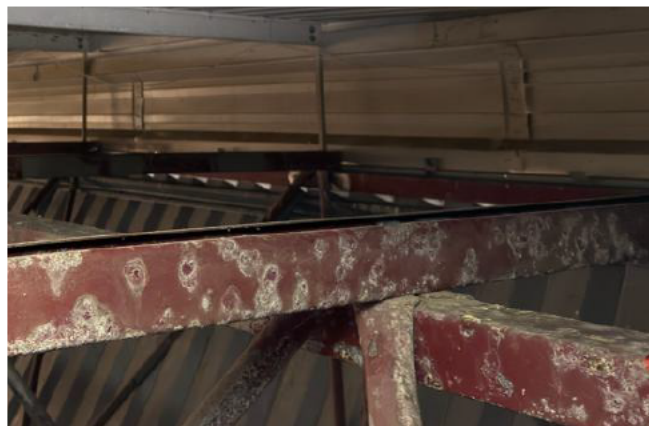
Photo 004 – Truss Top chord. Corrosion score 4.
