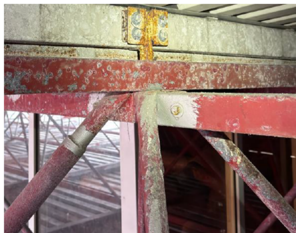
Photo 004 – Truss Diagonal. Corrosion score 4.
