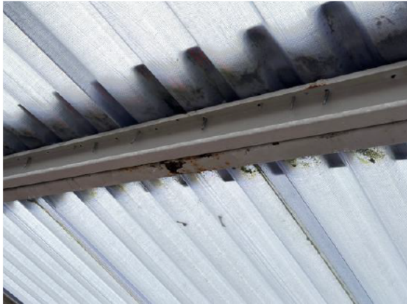
Photo 003 – Purlin corrosion. Corrosion score 4.
