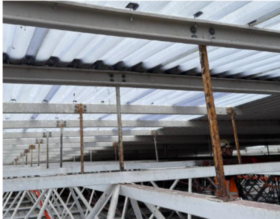
Photo 006 – Purlin Vertical Support Post northern side. Corrosion score 4.
