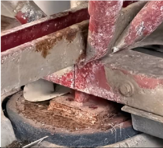
Photo 009 – Heavy corrosion between column and bottom chord. Corrosion score 4.
