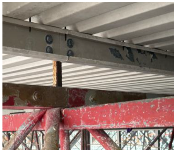
Photo 006 – Purlin corrosion. Corrosion score 2.
