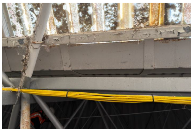
Photo 011 – Corrosion at intersection of upper and lower roof due to flashing at the corner. Corrosion level 4 on East side of the station.
