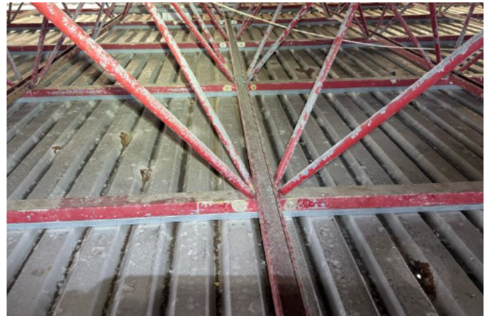
Photo 016 – Corrosion at the roof sheeting (Truss Level – Northern side).
