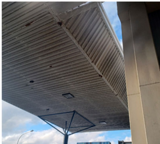
Corrosion at bottom roof sheeting corrosion score 3
