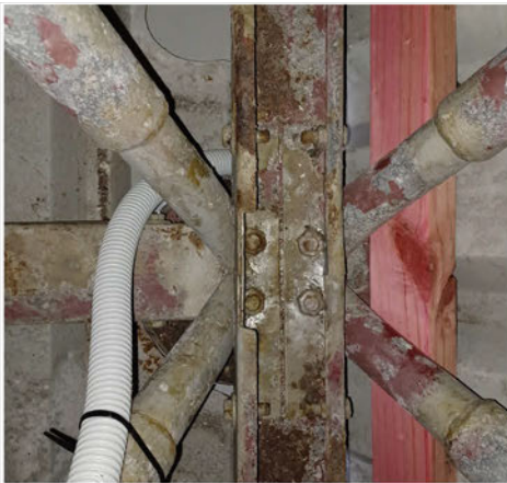
Bottom chord corrosion score 1
