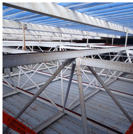
Top Chord and Diagonals
