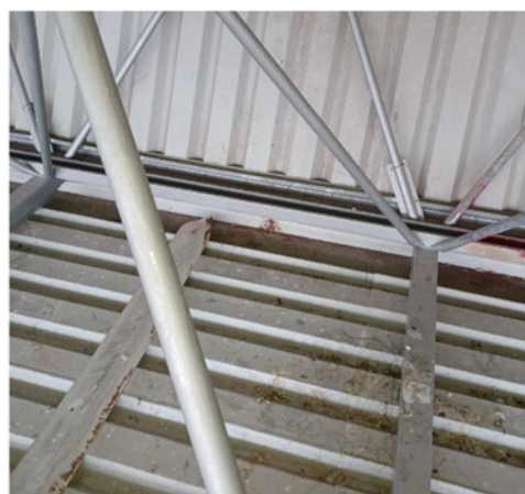
Holes in top roof sheeting
