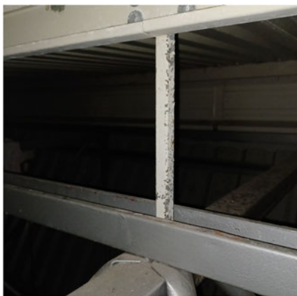
Purlin and SHS Support onto Top Chord
