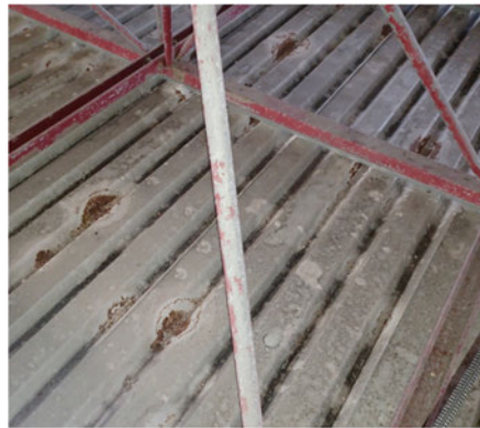
Corrosion at bottom roof sheeting corrosion score 4
