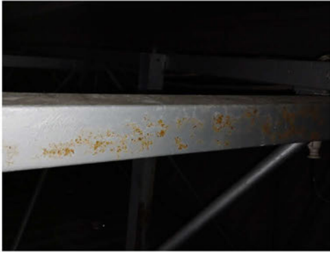
Truss top chord corrosion score 2
