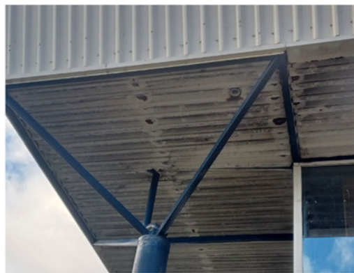
Corrosion at hold-down screws corrosion score 4
