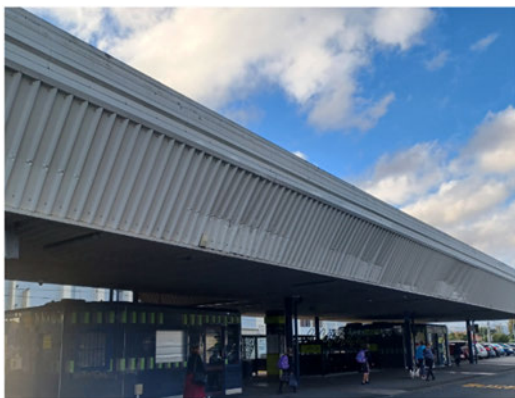
Corrosion at bottom roof sheeting corrosion score 3
