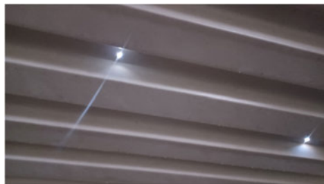
Holes in top roof sheeting
