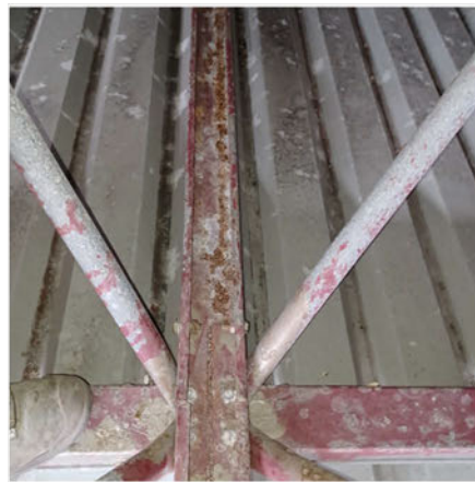
Bottom chord corrosion score 2
