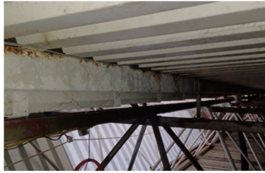
Corrosion at lower internal gutter corrosion score 4
