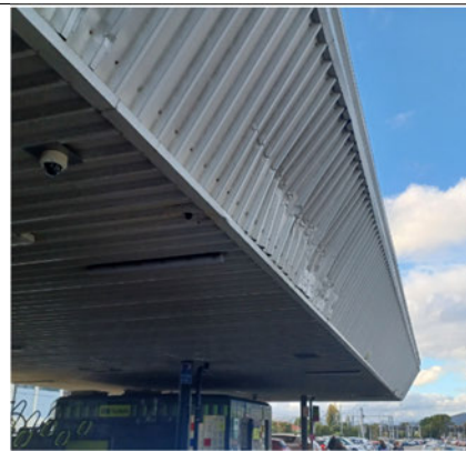
Corrosion at the intersection of upper and lower roofs due to flashing at the corner, corrosion score of 4
