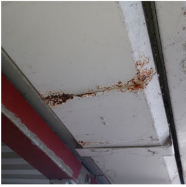
Corrosion at lower internal gutter corrosion score 4
