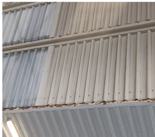
Corrosion at the intersection of upper and lower roofs due to flashing at the corner, corrosion score of 4
