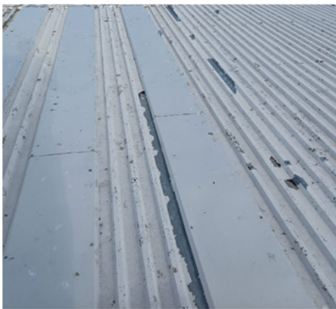
Corrosion at lower internal gutter corrosion score 4
