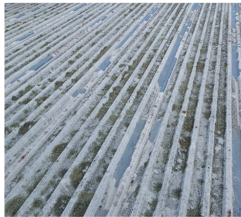
Corrosion at lower internal gutter corrosion score 4
