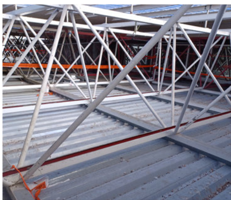
Bottom Chords and Diagonals
