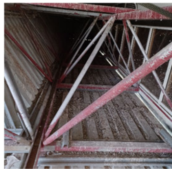
Corrosion at bottom roof sheeting corrosion score 4
