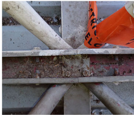
Bottom chord corrosion score 2
