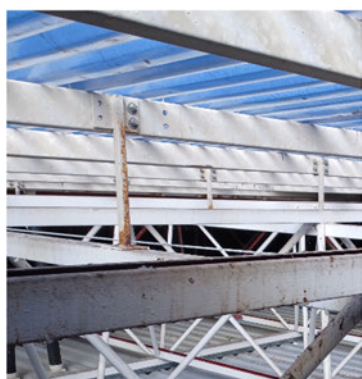
Corrosion spreading due to pipe fixings
