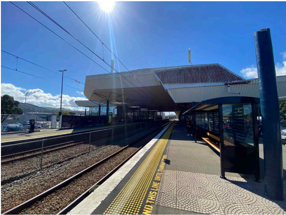
STATION RECEIVES GREAT SUNLIGHT IN SUMMER. STATION DOES NOT PROVIDE OPPORTUNITY TO ENJOY SUNSHINE, NOR WELCOMING SPACES TO SEEK SHADE.
