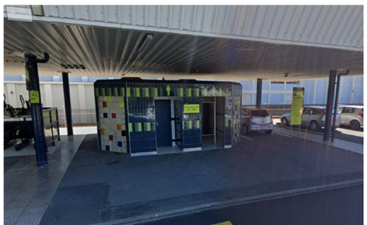
Existing toilet block with adjacent roof down pipes
