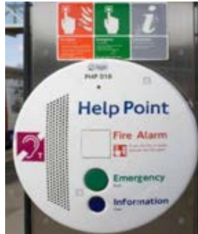
Figure 6-2: Typical PHP used in Metro/Railway environments
