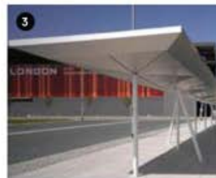
2 Platform Canopy Roof: A floating plane with thin edges, supported on elegant columns
