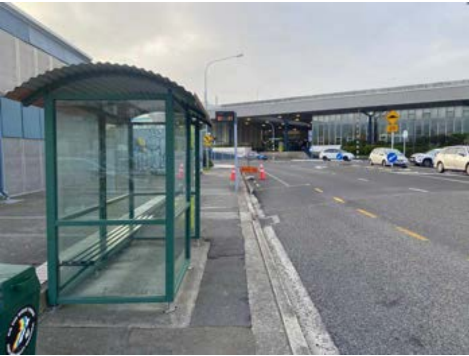
Figure 17: Photograph - Knights Rd - poor pedestrian and bus user infrastructure
