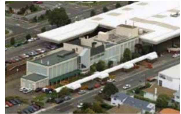
Figure 3 Waterloo Water Treatment Plant (source: WWL)
