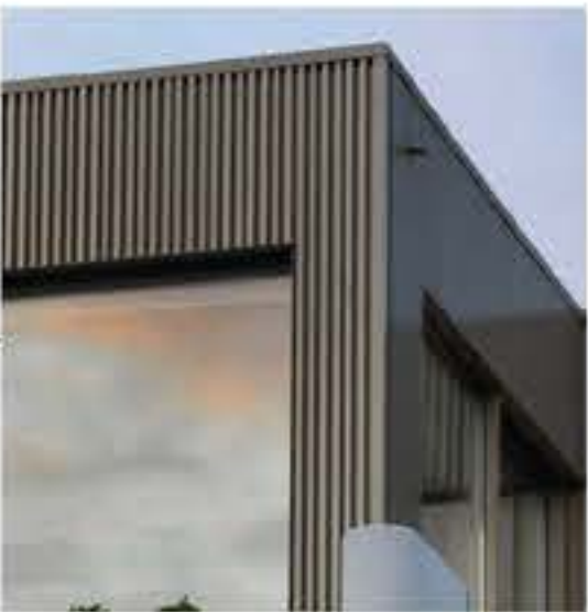
EWS-501 Aluminium cladding system
