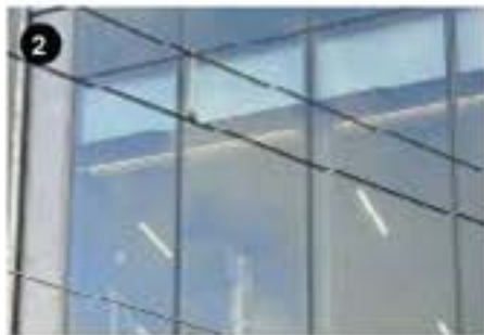
Unadorned glass facades provide a clean, easy to maintain surface that is durable.
