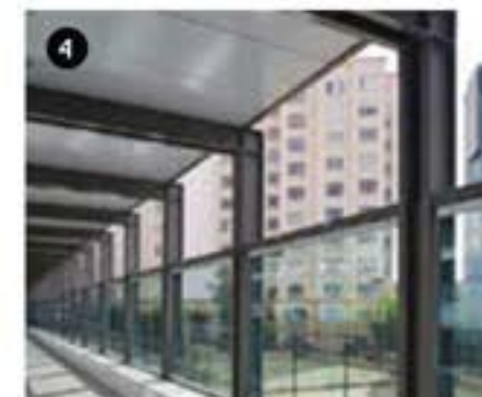
4 Glazed wind breaks provide protection from elements.
