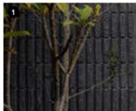
1 Wall Cladding: Ribbed block veneer provides solid, textured contrast to glazed waiting areas
