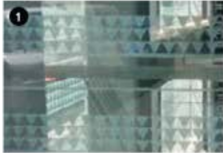
Ceramic frit applied to glass facade mitigate solar gain. Patterns can incorporate Māori Whenua design.
