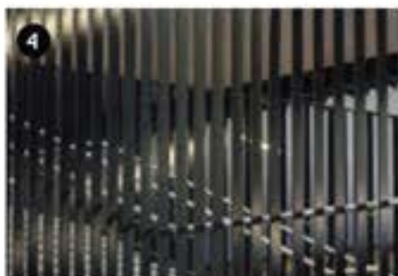
Battened ceilings can discreetly accommodate services and provide acoustic dampening.
