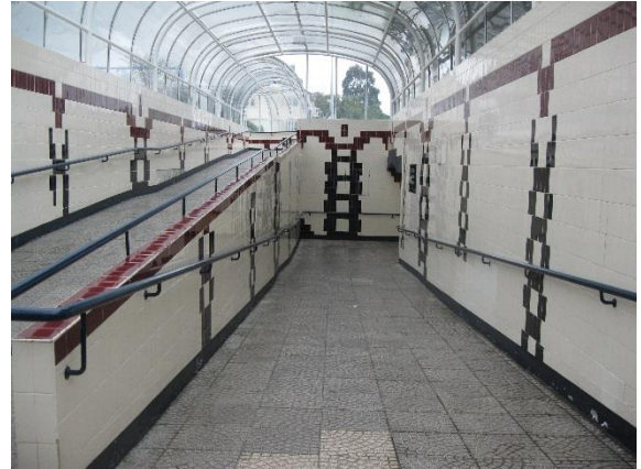
Photo 2 – Ramp Showing Cantilever Wall
